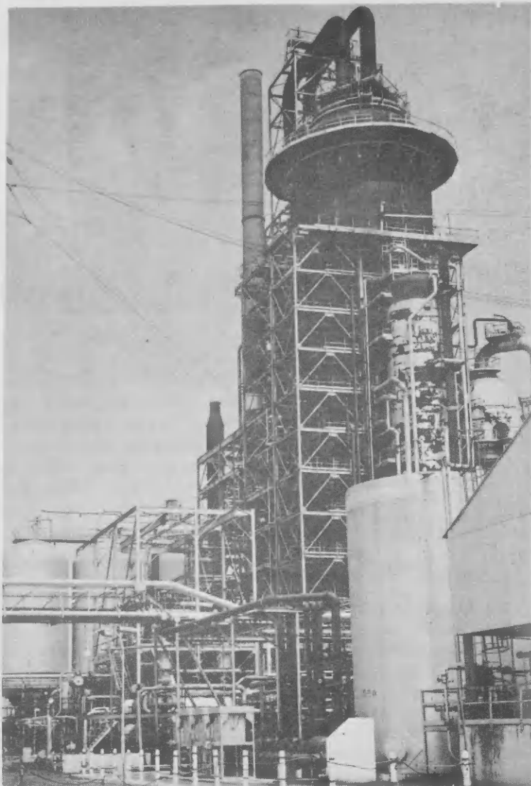
A streamlined PCAR returned to service March 30. Un PCAR renoba a bolbe na servicio Maart 30.
